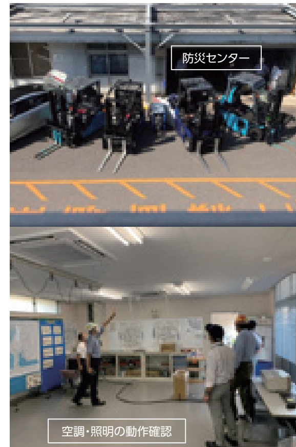
図9 防災センターへの給電 Fig.9 Power supply to disaster prevention center
